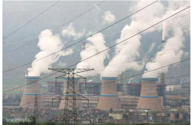
The state-owned, coal-burning Xuanwei Power Station in Yunnan province
